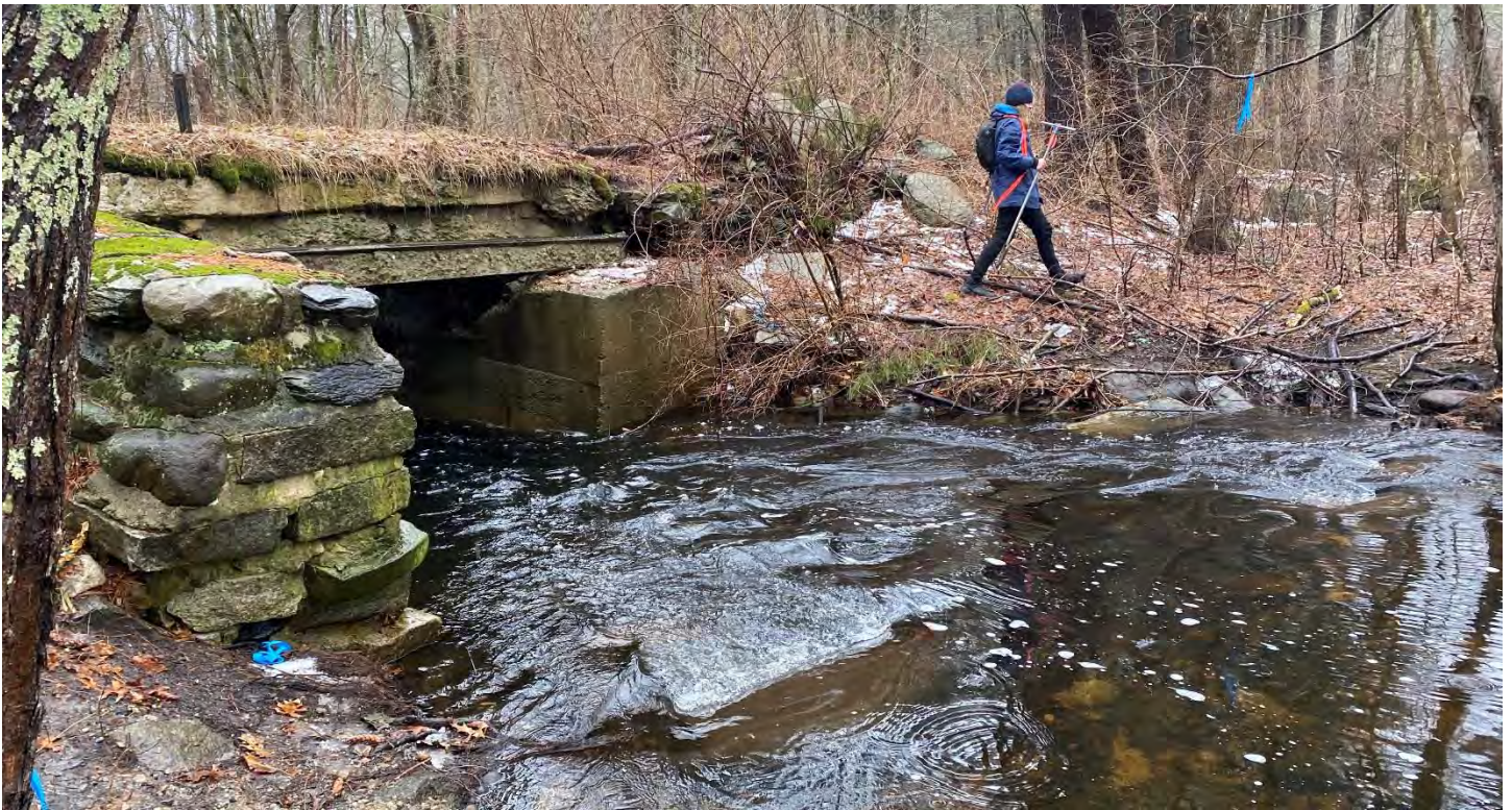
Photograph 6: Southwest view of Brandy Brow Road culvert from flag B-108.
