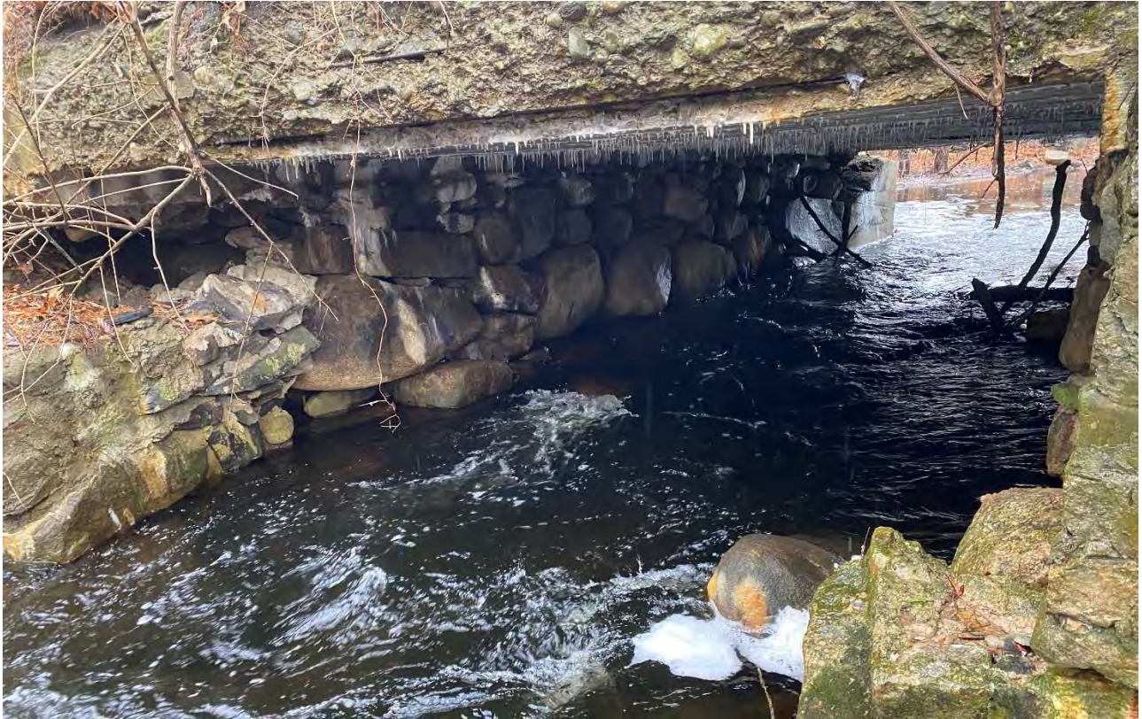
Photograph 8: North view of open-bottom-stone culvert beneath Brandy Brow Road.
