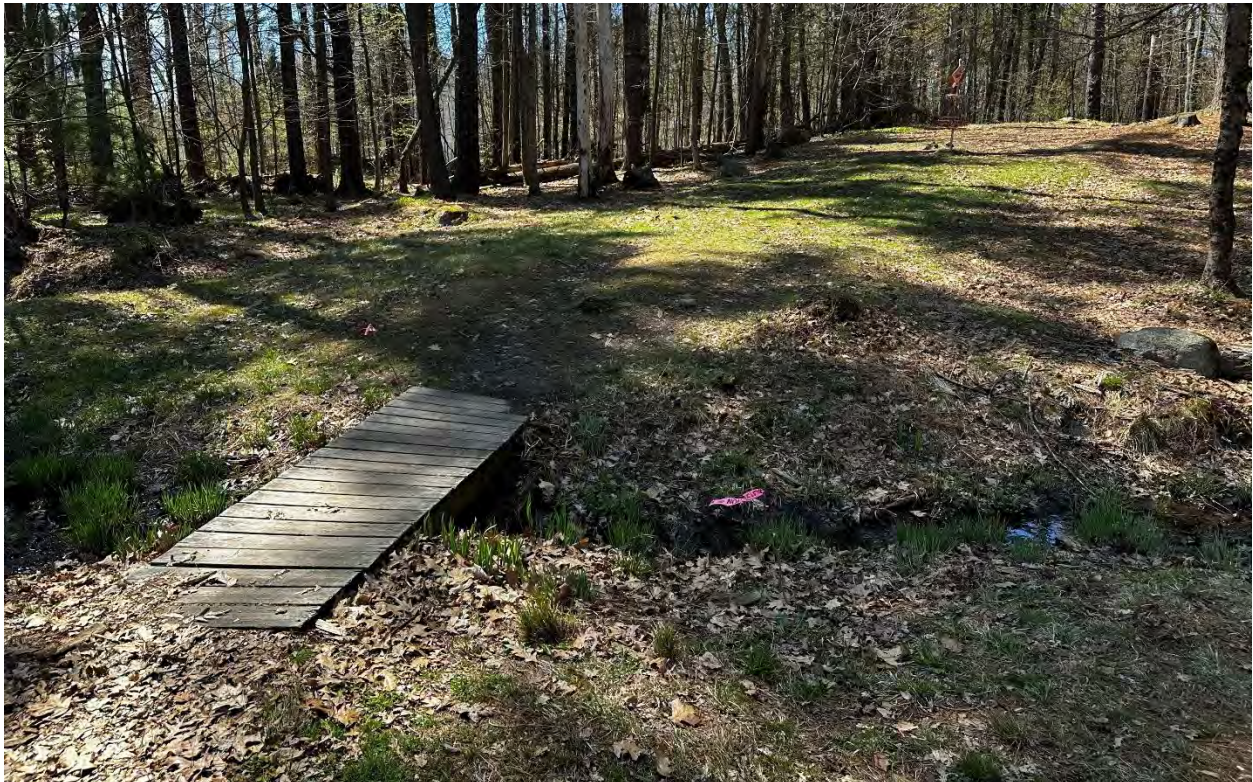
Photo 4: View of the existing timber footbridge spanning the intermittent stream facing southwest with the orange disc basket in the background. Pink flagging delineates the intermittent stream bank boundaries.
