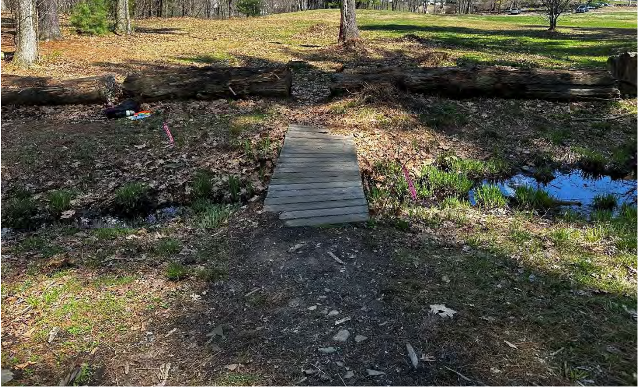
Photo 5: View of the footbridge facing northeast with the parking area in the background. The footbridge measures 10-feet long and 3-feet wide.
