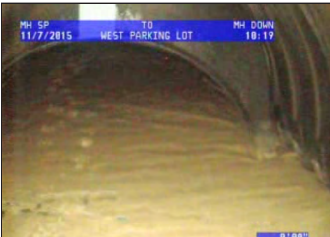
SEPARATOR ROW: Separator Row prior to cleaning
