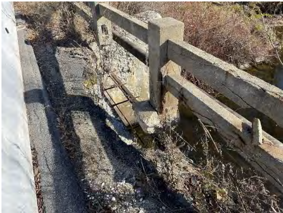
View of the current conditions of the deteriorating pavement and guard rail on the northern side of the Rosemont Street Bridge.
