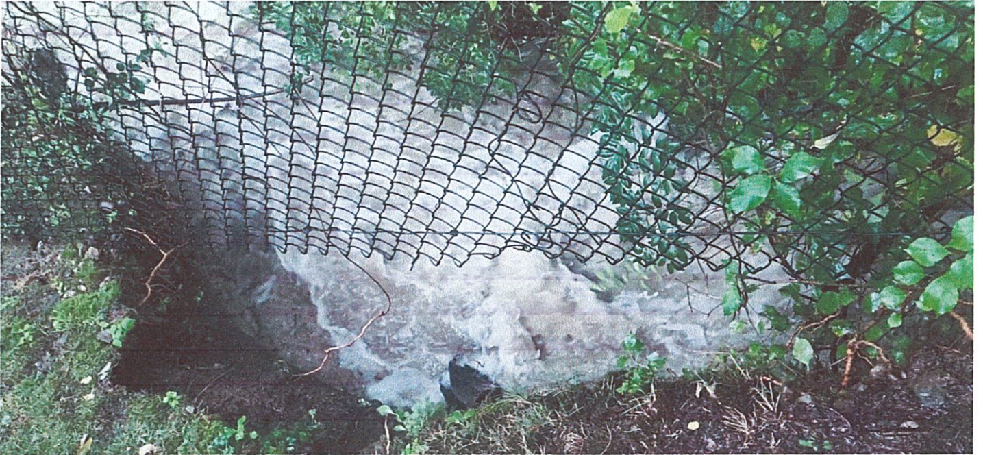
Water flowing through during the rain event.
