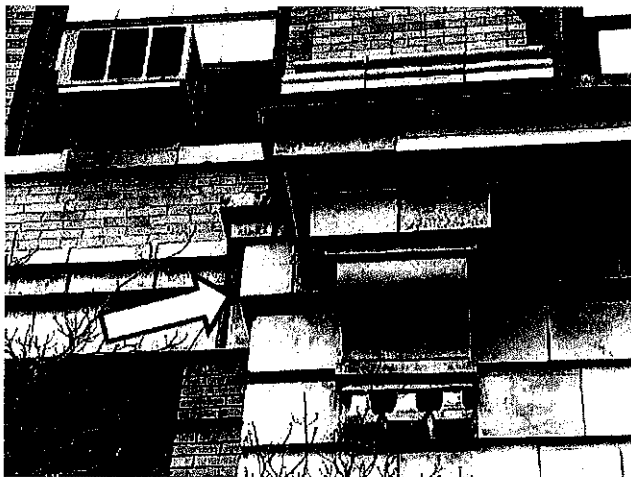
Photo 6 – Spalled/displaced stone feature on arched
