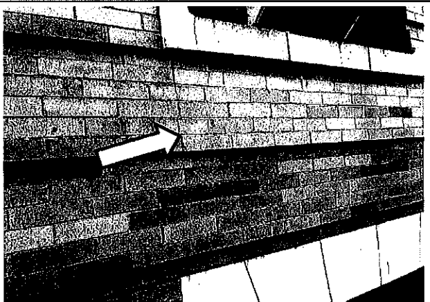
Photo 17 – Typical step cracked brick masonry
