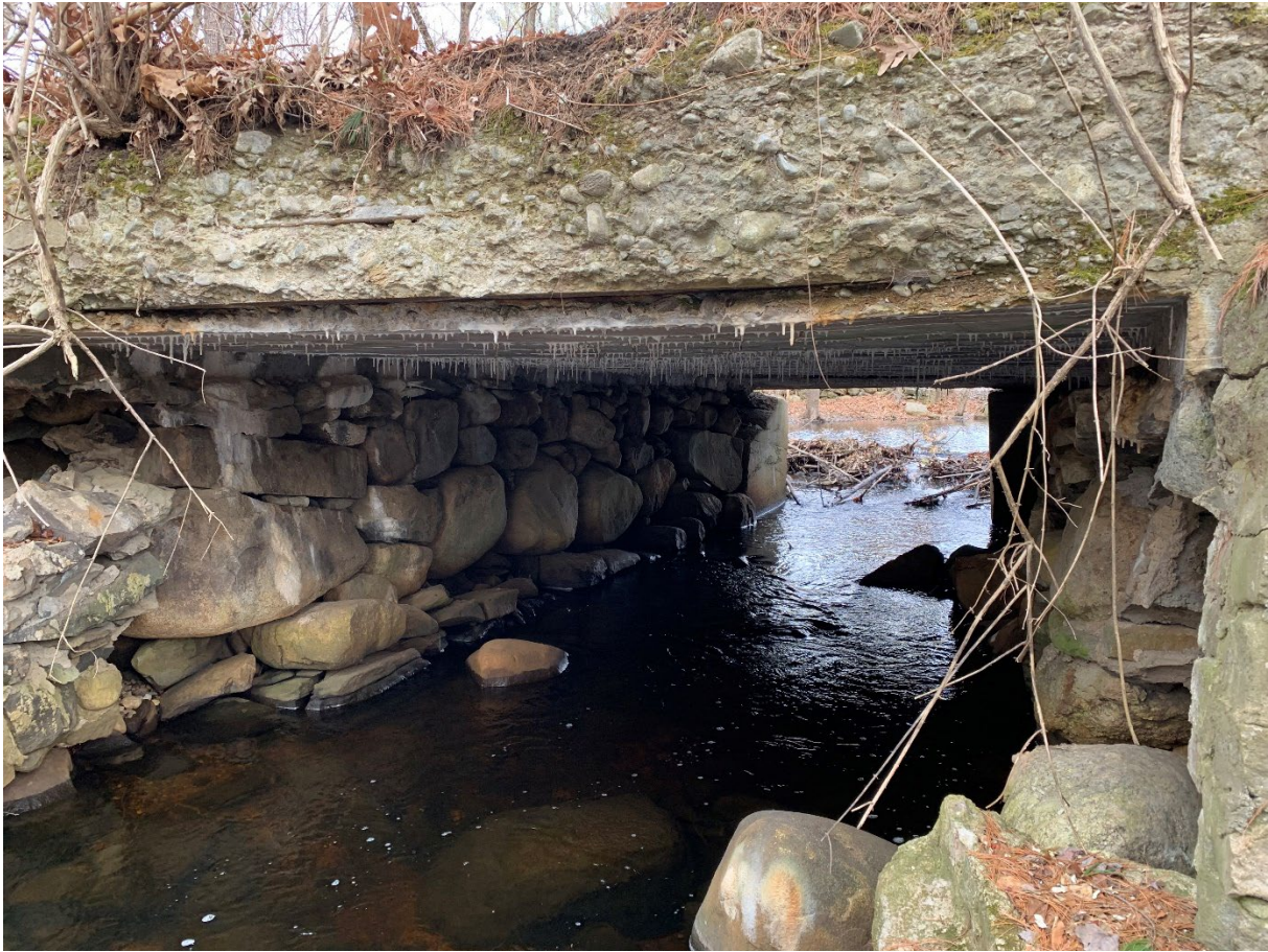
Inside Brandy Brow Road Culvert (Downstream)
