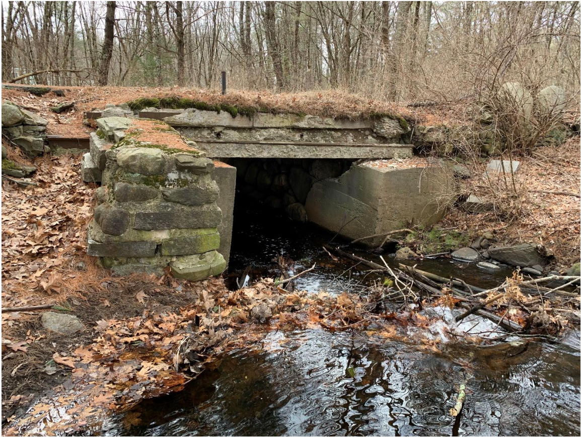
Brandy Brow Road Culvert (Upstream)
