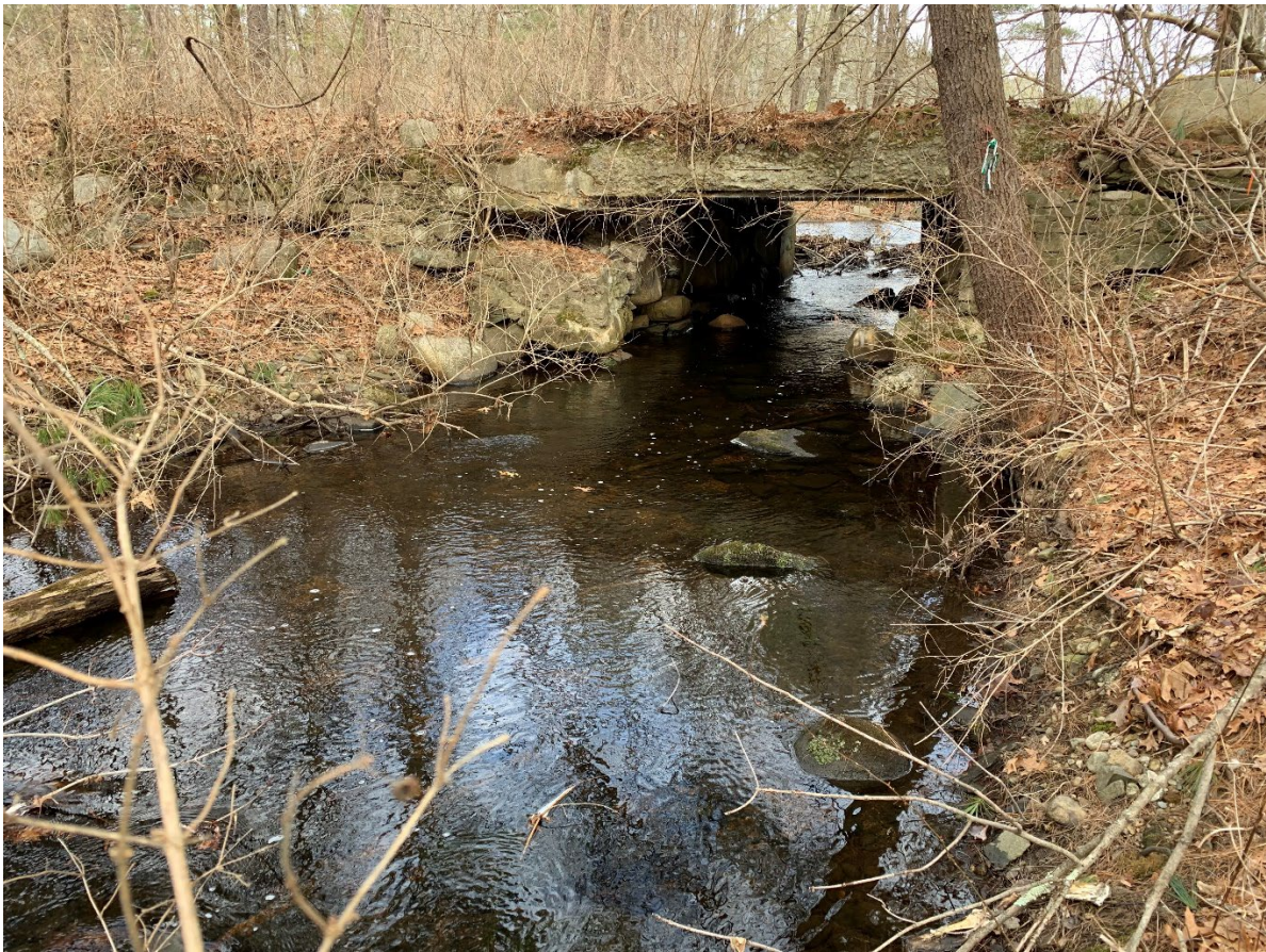
Brandy Brow Road Culvert (Downstream)
