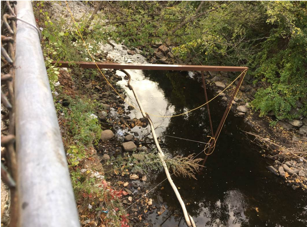
Photo 5: Attachment of containment boom ropes and support guy wires on day 3 (10/26/2016)
