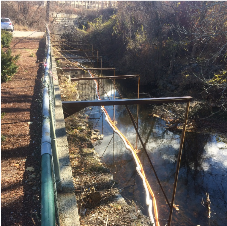
Photo 3: Semi-permanent containment boom on the Little River looking downstream (south). Photo taken 11/22/16
