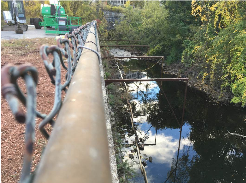
Photo 3: Containment boom supports installed on the first day of construction (10/24/2016)
