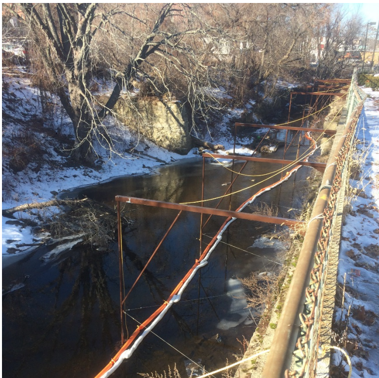
Photo 4: Semi-permanent containment boom on the Little River looking upstream (north). Photo taken 12/21/16
