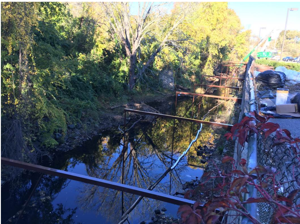
Photo 4: Containment Boom supports constructed on day 2 (10/25/2016) and work beginning on day 3 (10/26/2016), new temporary sorbent boom sections are pictured near the center of the photo
