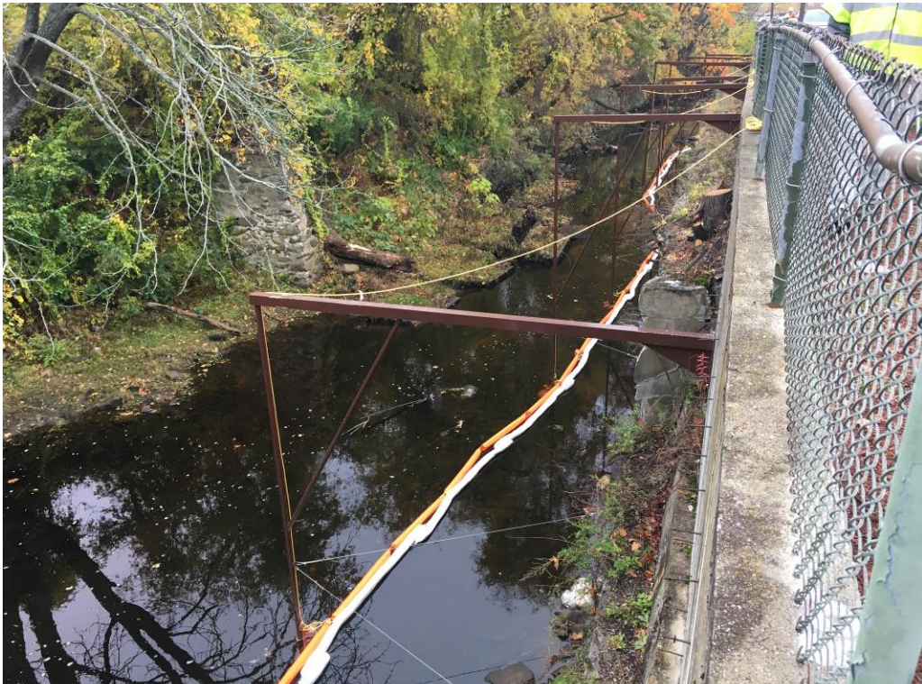
Photo 6: View of the completed boom installation facing north/upstream.
