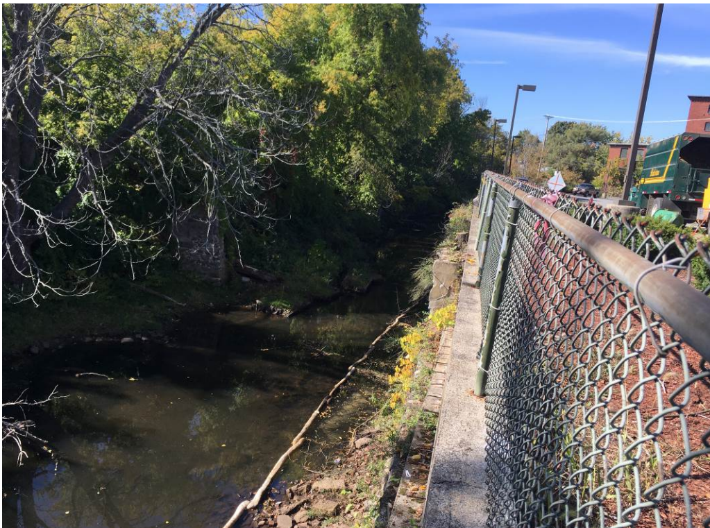
Photo 2: Retaining wall and temporary sorbent boom after vegetation clearing (10/12/2016)
