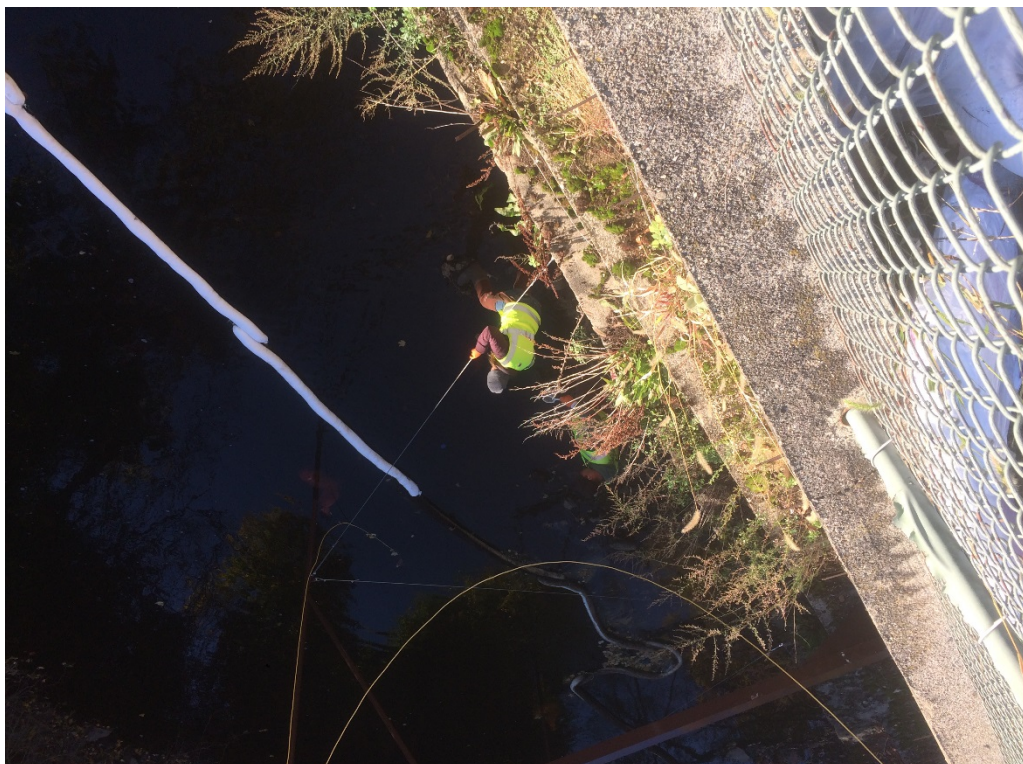
Photo 2: Temporary containment boom on the Little River during construction of semi-permanent containment boom system. NAPL sampling shown being performed by GZA. Photo taken 11/1/16
