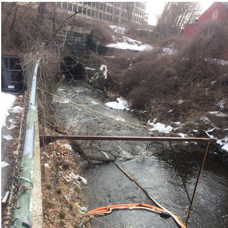
Photo 8: Southern end of semi-permanent containment boom on the Little River, looking downstream (south). Fallen tree visible on temporary boom "tail". Photo taken 2/24/17
