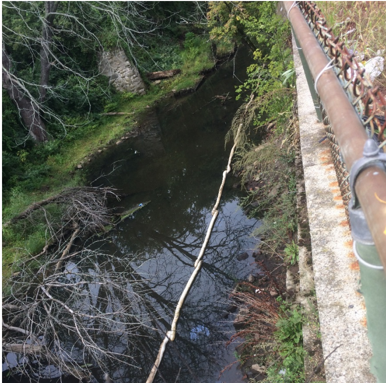
Photo 1: Temporary containment boom on the Little River looking upstream (north). Photo taken 9/27/16
