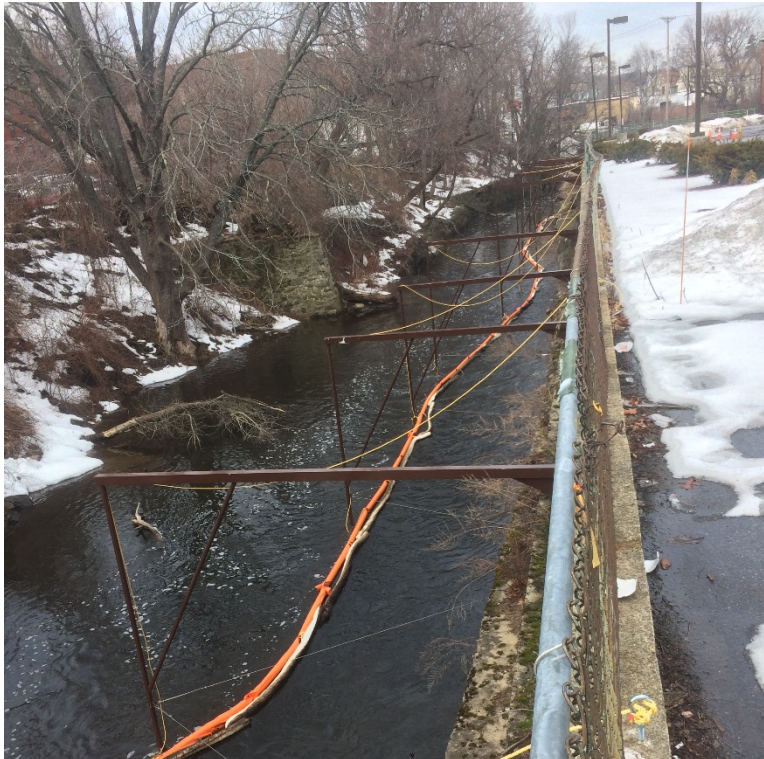
Photo 7: Semi-permanent containment boom on the Little River looking upstream (north). Photo taken 2/27/17
