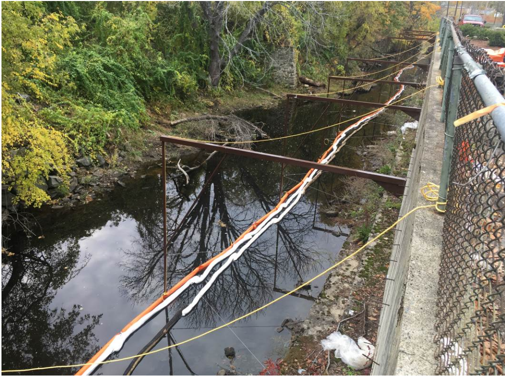
Photo 3: Curtain boom and new sorbent boom installed. Spent temporary sorbent boom shown pending removal.
