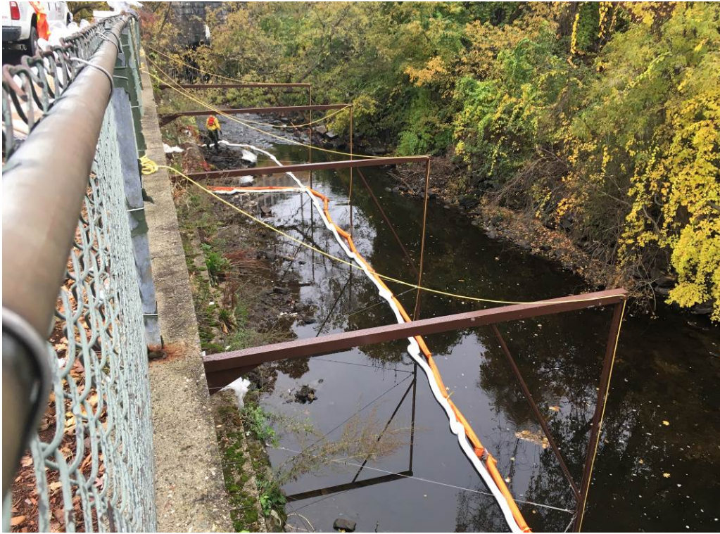
Photo 5: View of southern/downstream end of the boom containment system. Temporary sorbent boom extends beyond the retaining wall and boom supports to the south.
