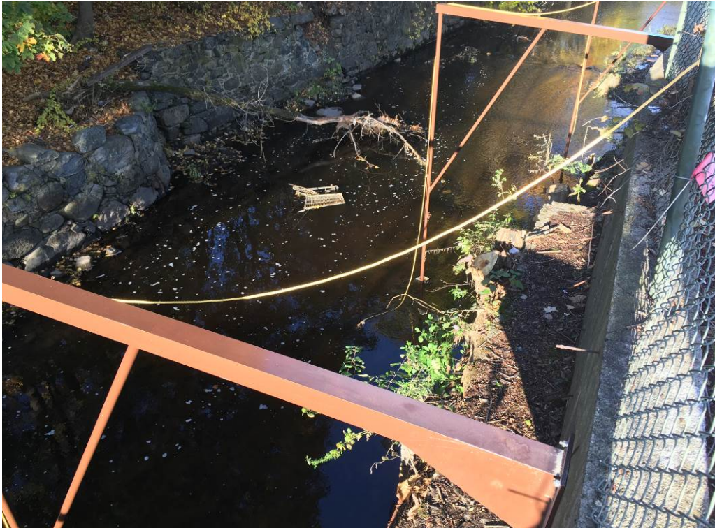
Photo 1: Northern containment boom supports prior to guy wire installation.
