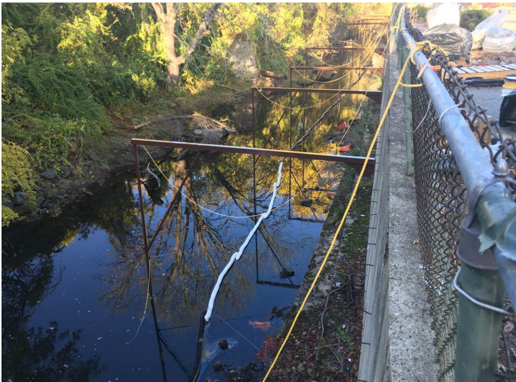
Photo 2: Guy wire installation complete for all supports. Temporary sorbent boom pending replacement.
