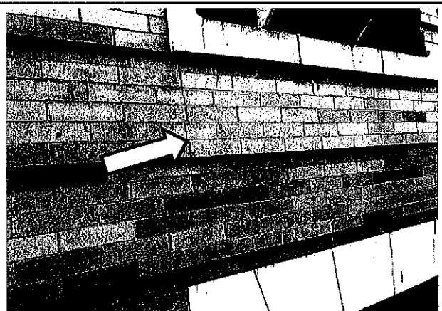
Photo 17 – Typical step cracked brick masonry
