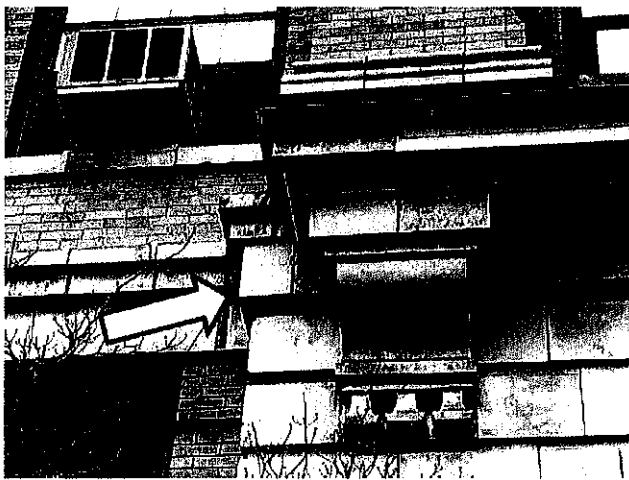
Photo 6 – Spalled/displaced stone feature on arched
