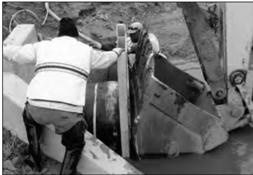
Pallet Push method for installing CheckMate® Valve
