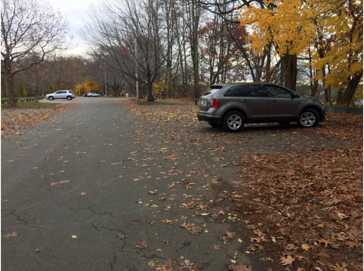
Photo 1: Easterly view of southern parking area. Existing pavement on the south (right) side of the parking area will be converted to a walkway. New wood guardrail will be installed between the parking area and walkway, and a new ornamental fence will be installed between the walkway and river. Parking area will be re-stripped.
